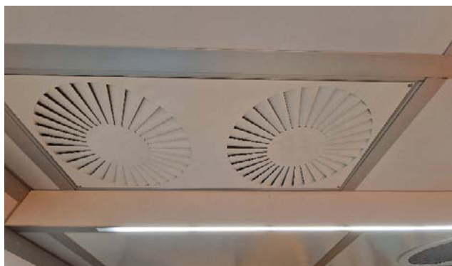
Left: FFU with swirl plate. Right: Power vs. air volume speed for a FFU with and without swirl plate.
